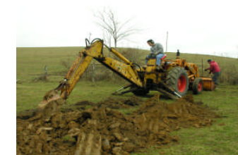
Nigel & Dale work on a spring development to bring water to the cows in the new rotational grazing system.
